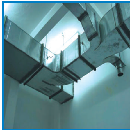
CEI-EX04 GI DUCTING SYSTEM
